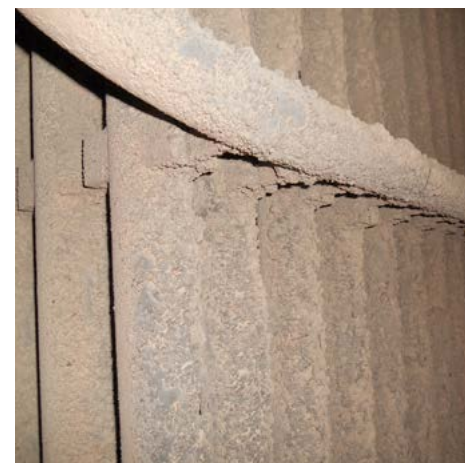
Tube attachment welds which are encrusted with debris. Neither visual inspection nor NDT are possible in this condition
