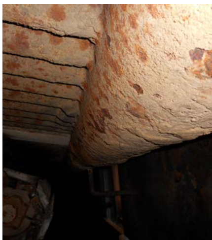
Header tube stubs prior to preparation for inspection and NDT
