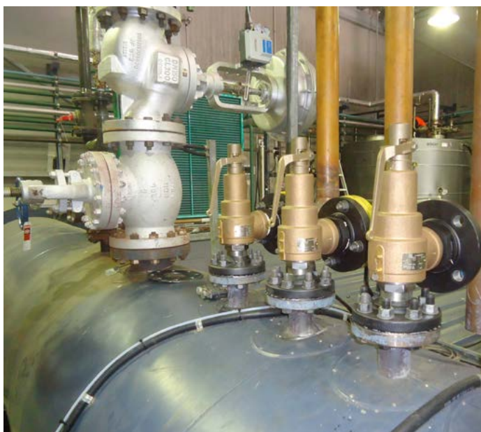
TAYLOR Safety Valves installed on saturated steam boiler main drum (Australian photo courtesy JPS Valves & Service Pty Ltd)
