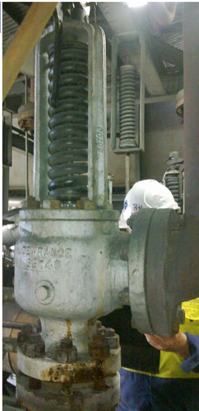
DEWRANCE Safety Valve installed on main steam drum in a power station. The valve was 55 years old and still in service (Australian photo courtesy JPS Valves & Service Pty Ltd, see article page 12)
