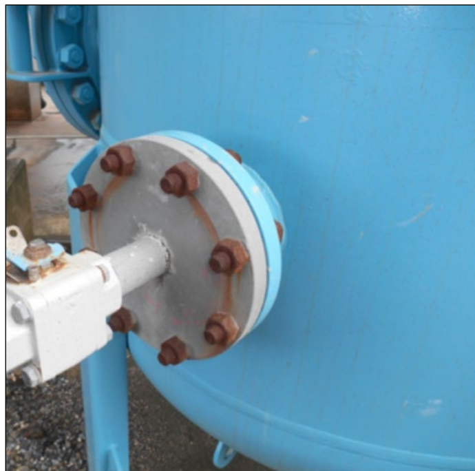
Unpainted flange bolting at a large air receiver
