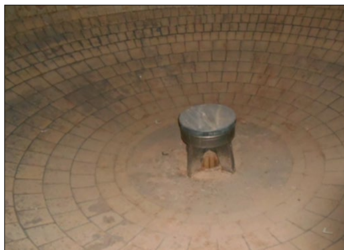
Figure 4. Floor area of a large process vessel showing typical internal ceramic lining installed for erosion and chemical attack
