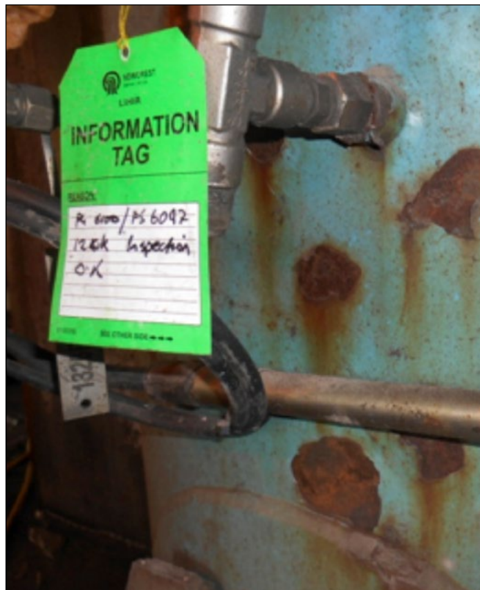
Air receiver showing degradation of external protective coating most likely due to impact damage or poor coating application
