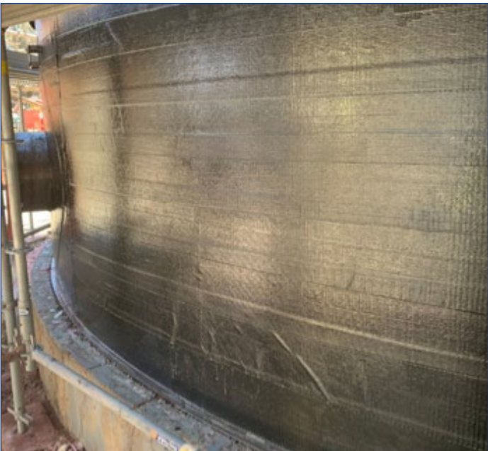
Figure 1. Composite wrap system curbs corrosion under insulation at nickel mine
