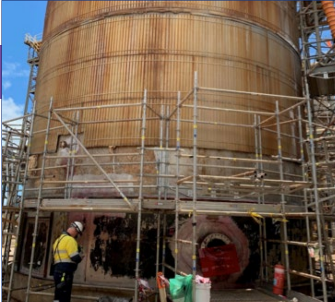
Figure 2. Stainless steel feed tank repaired and protected with Belzona SuperWrap II
