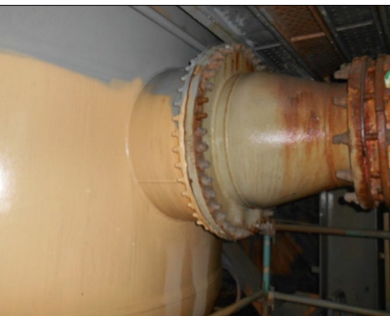
Figure 6. A large process vessel after repair to failed protective coating. The associated reducer was removed and re-coated while piping downstream was replaced
