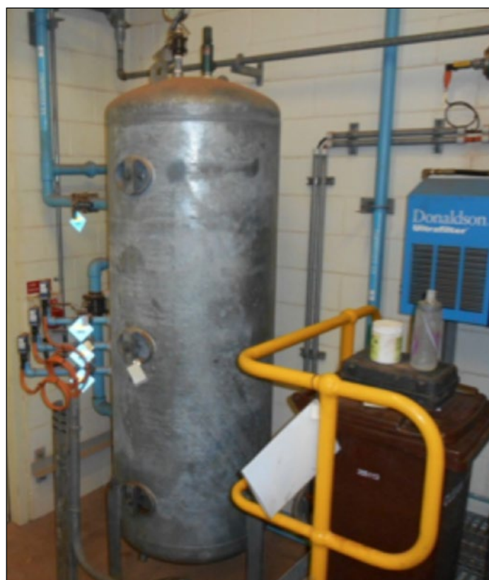
Figure 2. Galvanised air receiver beginning to show deterioration due to sacrificial oxidation of the galvanising zinc
